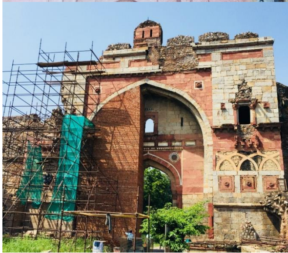
'Figure 2,; Conservation work at Sher Shah Gate
